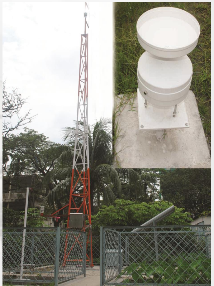
Automatic Weather Station at Atmospheric Observatory, DoM
