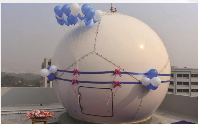
Satellite Ground Station at DoM, DU
